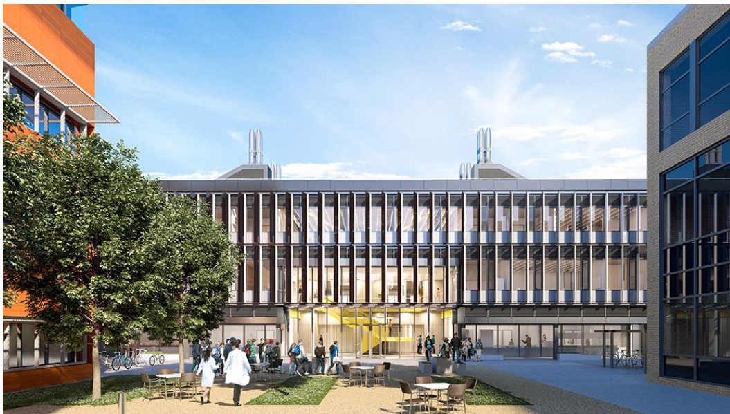
Figure 1: New civil engineering building
