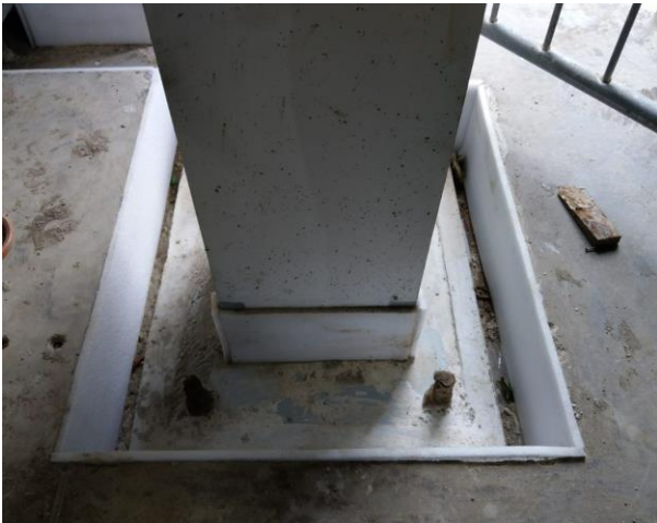
15. DfD column baseplate detail
