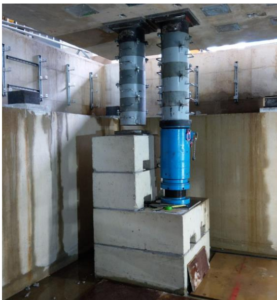
19. Hydraulic jack to lower strong floor into position.
