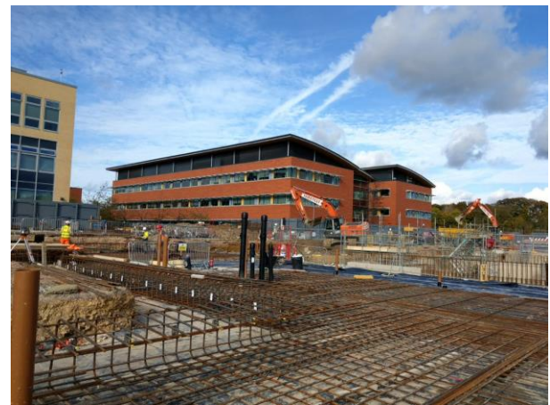
7. Basement and ground floor reinforcement
