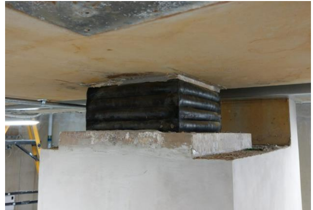
20. Strong floor elastomeric bearing
